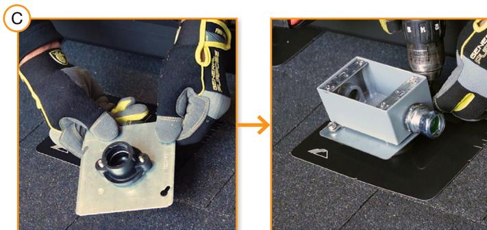
To prevent corrosion and roof staining, cold galvanizing compound should be applied to any holes drilled through galvanized steel.
